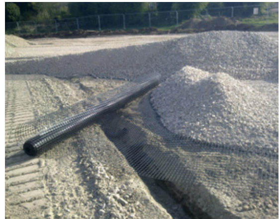
Plastic mesh within stone layer
