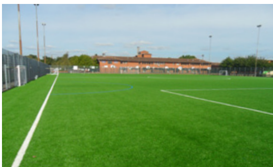
Resurfaced pitch with 60 mm pile 3G long pile onto a 15 mm shock pad for football and for rugby training
