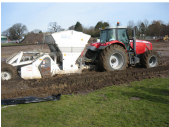
Installation of ground stabilisation treatment
